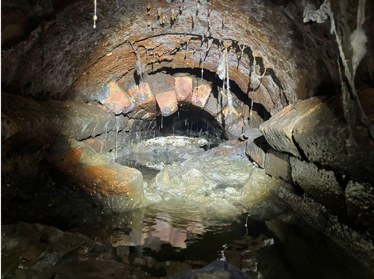
A Victorian sewer under the Shore Road in north Belfast.
